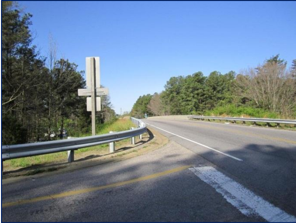
Photograph 5: I-95 Northbound Ramp at Rives Road – Looking to the West
