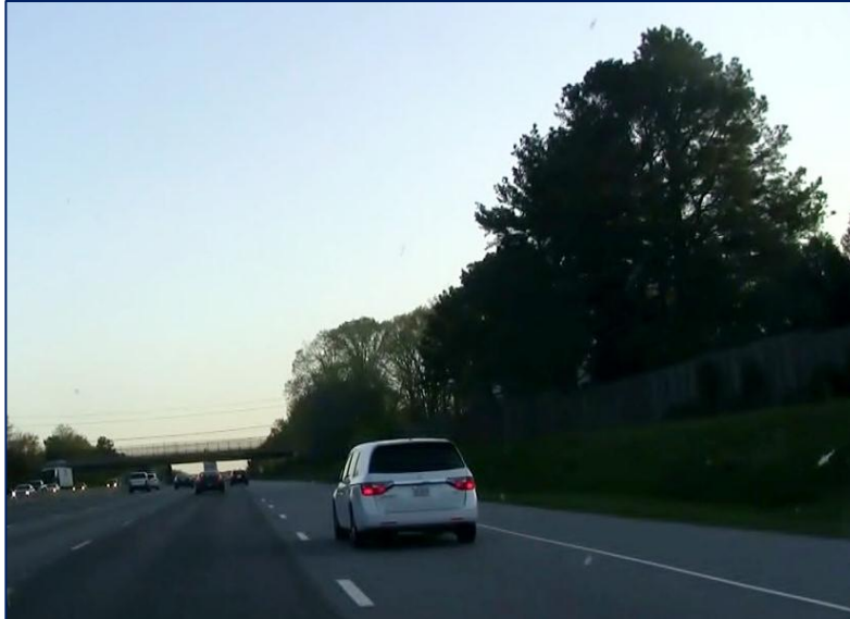
Photograph 4: End of Northbound Temple Avenue Acceleration Lane (Northern On-Ramp)
