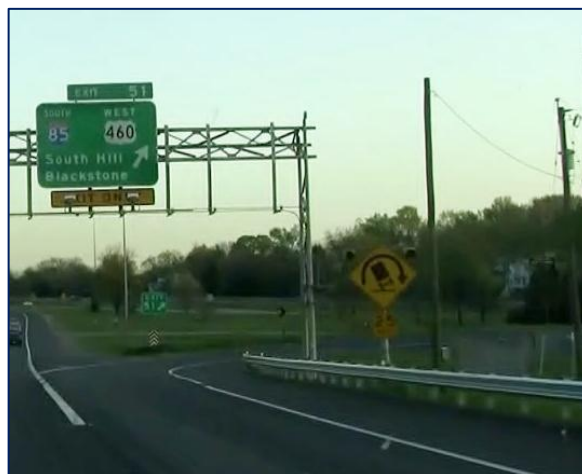
Photograph 3: Continuous Flashing Beacons on Truck Rollover Warning Sign
