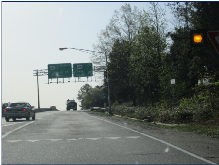
Photograph 10: Northbound I-85 to Southbound I-95 Weave
