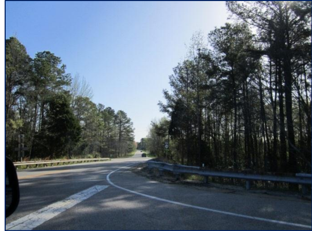
Photograph 6: I-95 Northbound Ramp at Rives Road – Looking to the East
