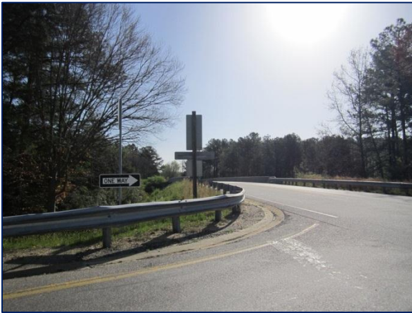
Photograph 7: I-95 Southbound Ramp at Rives Road – Looking to the East
