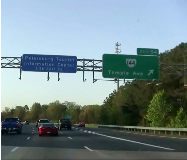
Located at MP 54.3
