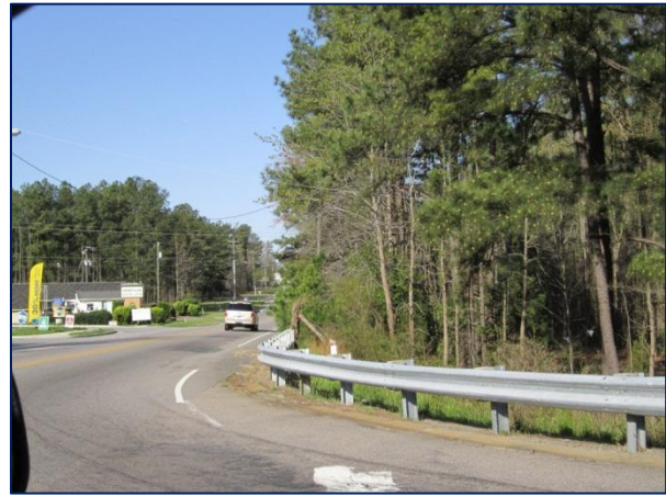
Photograph 8: I-95 Southbound Ramp at Rives Road - Looking to the West
