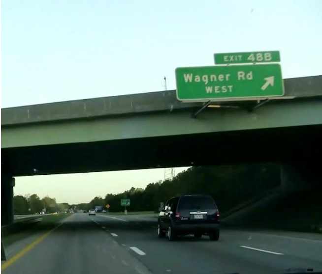
Located at MP 48.7
