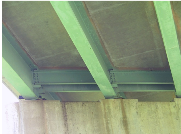
Photo 9: Guano staining on side of pier**
